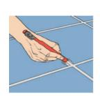
e. Any light haze remaining on the tile surface can be cleaned off the next dy using the EMULSIFYING PAD & GRIPPER and an alkaline detergent. Do not allow the haze to remain on the surface for any longer than 24 hours.
